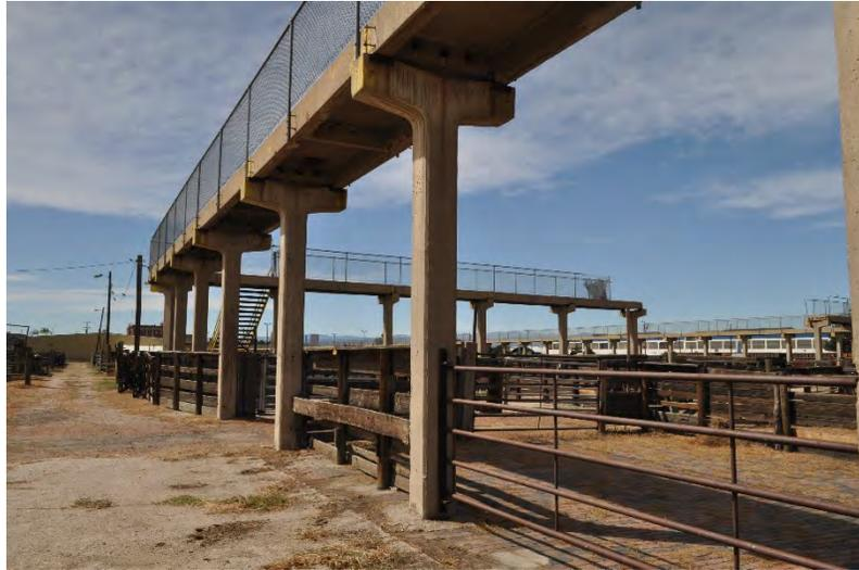
**Brief description:** Concrete columns and platform, metal stairs and chain-link fence comprise the catwalks. They have 20-24-foot tall t-shaped columns that are 1'x1' in diameter and 5' wide at the top (t-shaped top extension). The concrete contains remnants of yellow paint. The walk is fenced with a 4-foot tall chain-link fence. Metal grated stairs provide access at certain points. Some catwalk segments have been repaired and others have collapsed.
