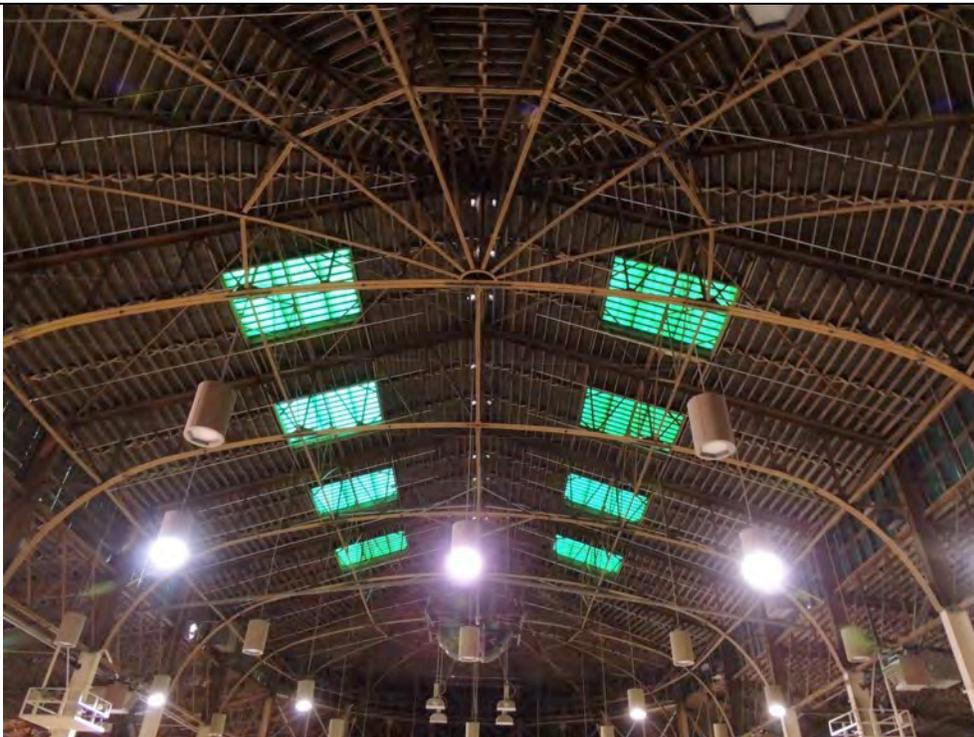
Steel roof trusses and skylights. Clerestory is covered, 2016.
