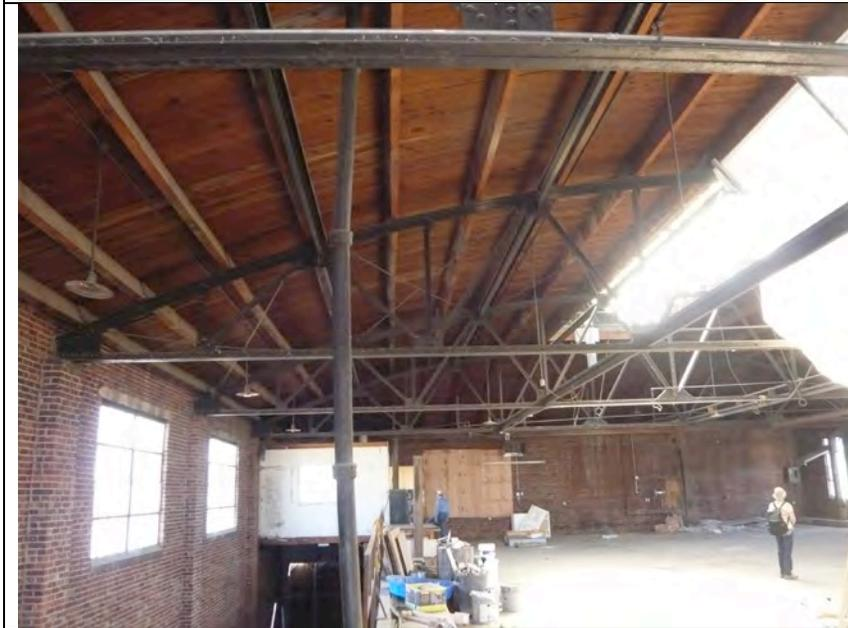
The upper floor of the interior is lofted providing a dramatic clear span. The space is crowned with exposed bowed steel trusses and an operable clerestory that lights and ventilates the space.
