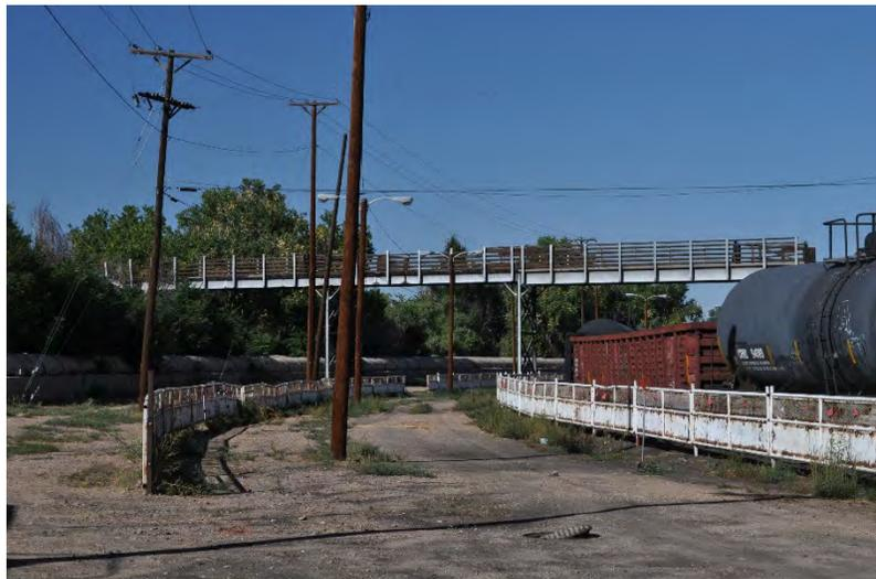
concrete base support five approximately 80-foot steel spans. The 9-foot wide deck consists of three concrete approach spans on the east side and wood decking extending to the western end of the structure. A railing lines the entire bridge (including inside the two pony truss spans), with steel railings bolted to the deck. Six slats of wood are attached to the posts.
