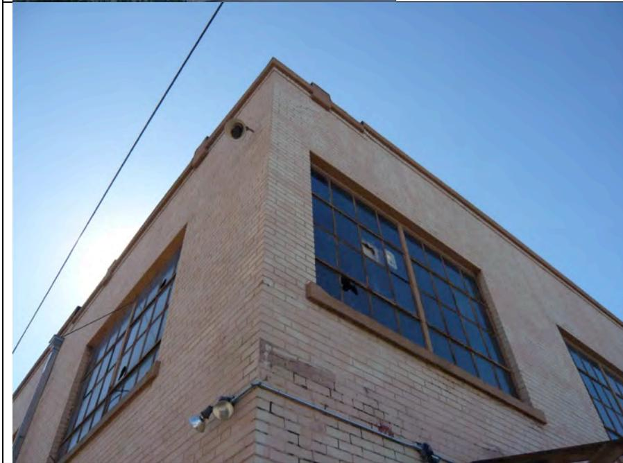
Detail of steel warehouse windows. Some ganged glazing panels are operable awnings.
