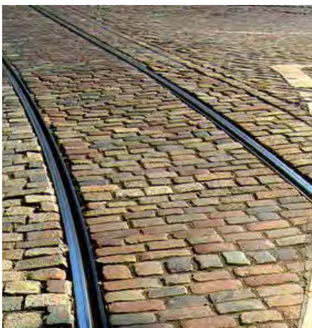
Decorative metal inlays such as re-purposed rails can add to the narrative and character of the Campus.
