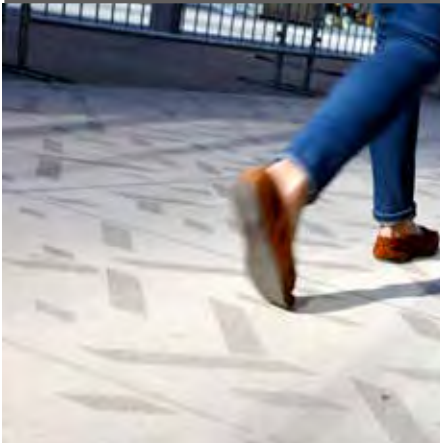
Standard concrete with decorative finishes and integral colors at Key Intersections.
