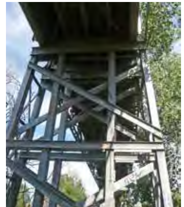
The historic sheep bridge
