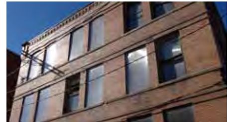
Preserve the ratio of window openings to solid wall on a primary facade.
