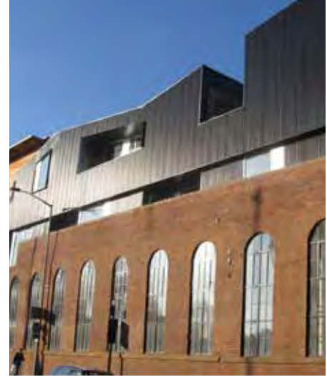
For a larger addition, break up the mass of the addition into smaller modules.
