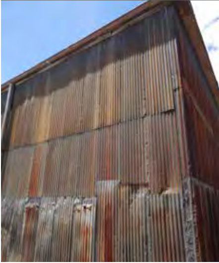
Preserve original building materials, where feasible.
