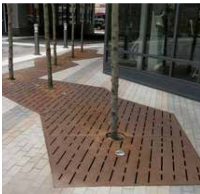
Tree trench filters are tree planting areas, often covered with a grate, that include large underground areas with materials that store and filter stormwater
