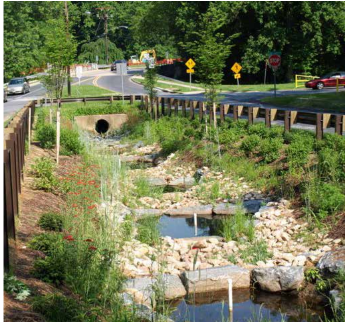
Open swale conveyance channels allow water to move across the site in a natural setting that increases water infiltration.
