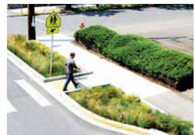
Infiltration planters are bioretention areas with deeper above ground containers to allow water to sit and slowly filtrate and infiltrate
