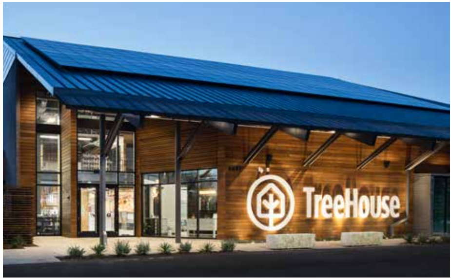
Consider accommodating large scale signage on buildings intended for public use, such as arenas.
