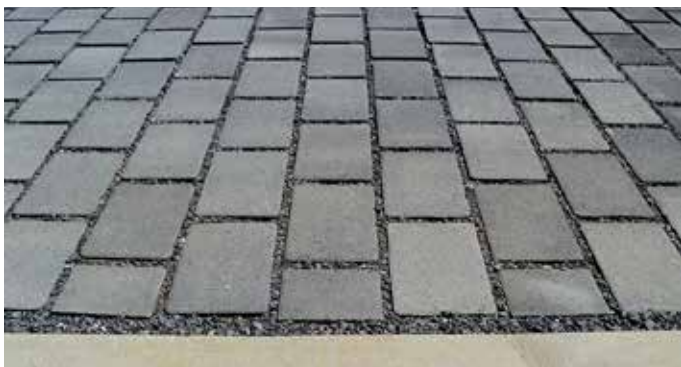
Permeable paving systems allow water to pass around pavers and infiltrate into the soil, reducing runoff and filtering stormwater.
