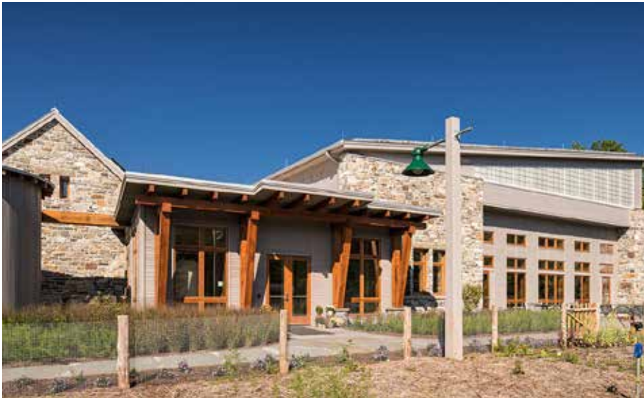
Ground floor wall offsets provide relief at the pedestrian level to avoid a long wall.
