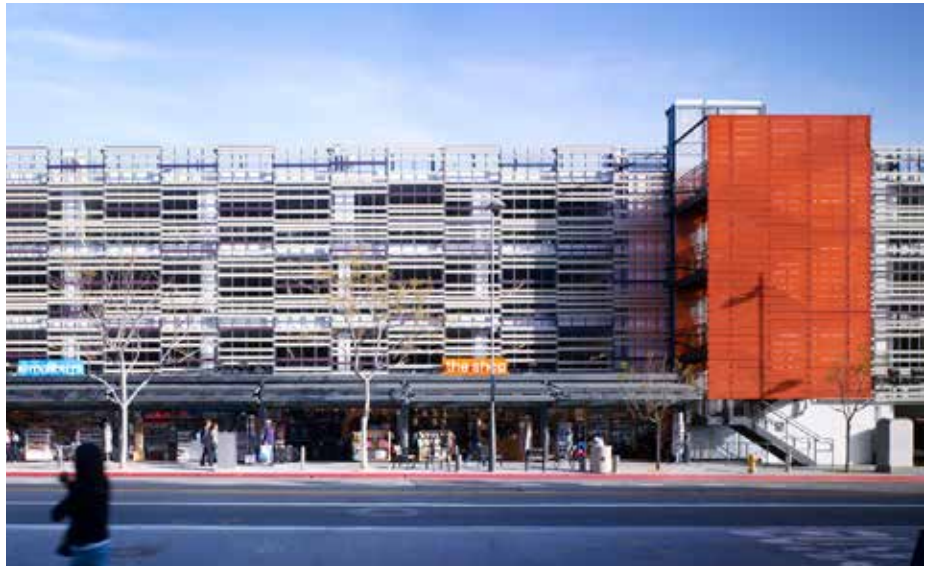
Design parking structures to limit the view of parked cars and angled ramps from adjacent pedestrian-oriented public spaces.
