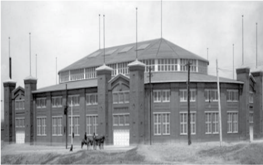
The 1909 Stadium Arena is a treasured historic building and was designated a Denver Landmark in 2016.
