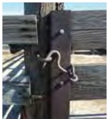
NWC: Metal gate gusset and latch
