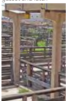
NWC: Historic "T construction" concrete catwalk posts
