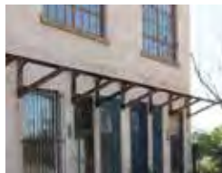
NWC: Metal awning brackets
