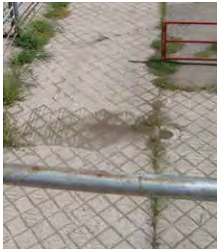
NWC: Concrete paving
