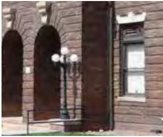
NWC: Traditional lighting
