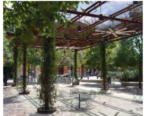
Level 3 Example, Pearl Brewery District, San Antonio. Historic metal screen reused as a canopy shade structure
