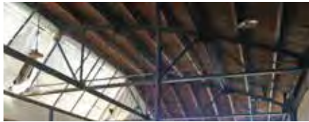
NWC: Historic steel truss roof structure
