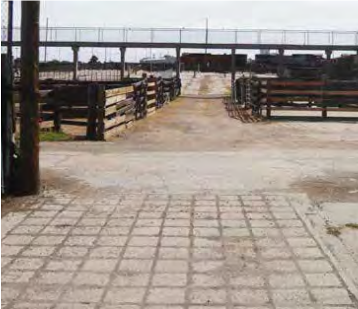
NWC: Concrete paving
