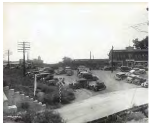
Area east of the railroad at Wards Hotel, 1934
