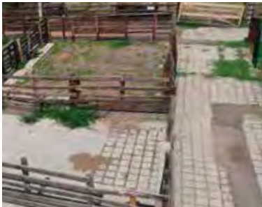
NWC: Brick and concrete paving defines the pens from the walkways in the Yards
