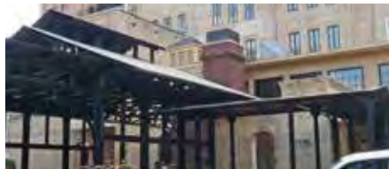
Pearl Brewery District: Metal framing used in a roof structures
