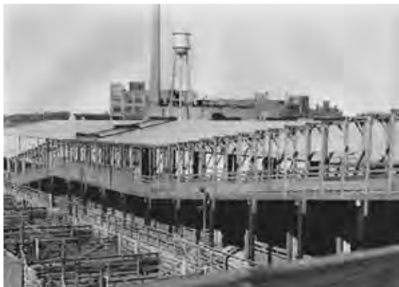
Stock overpass on east side of Sheep Barn; c. 1952
