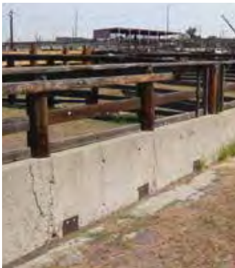
NWC: Concrete stem wall with metal gussets and wood frame railing
