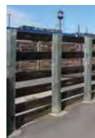
NWC: Concrete and wood posts
