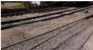
NWC: Historic rail lines run along National Western Drive and behind the Artist Studios
