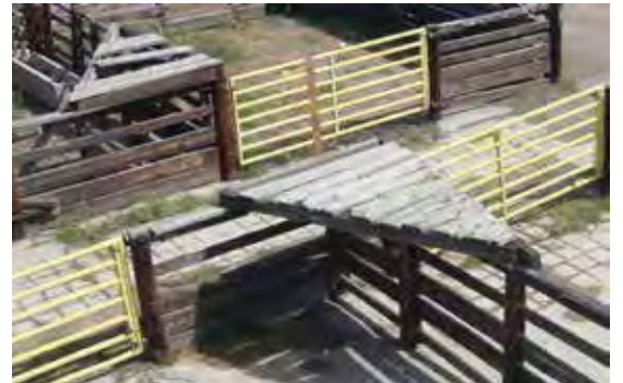
NWC: Wood and metal pen structures; concrete paving
