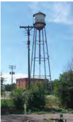
NWC: View of the historic Armour water tower
