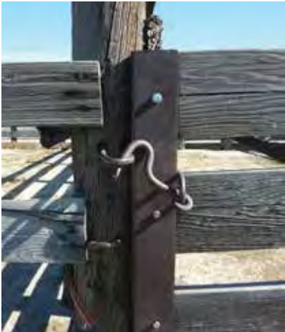
NWC: Wood and metal gusset pen structure
