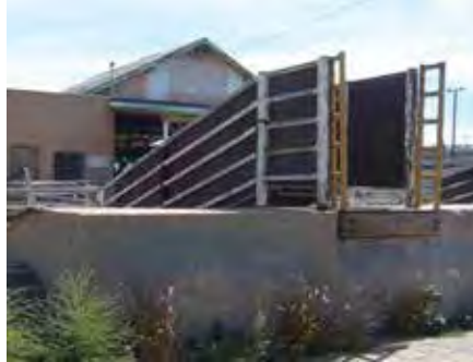
NWC: Concrete and metal loading ramp
