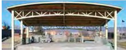
Prescott Valley: Metal trusses used in the roof structure of a performance space
