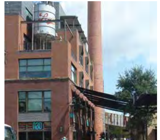
Pearl Brewery District: A historic smokestack and tank are reused as aesthetic elements
