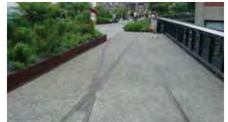
The High Line: Rail lines embedded in walkway reflect the historic rail circulation pattern
