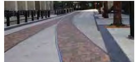
Minneapolis: Rails are highlighted with brick pavers to reflect historic circulation patterns
